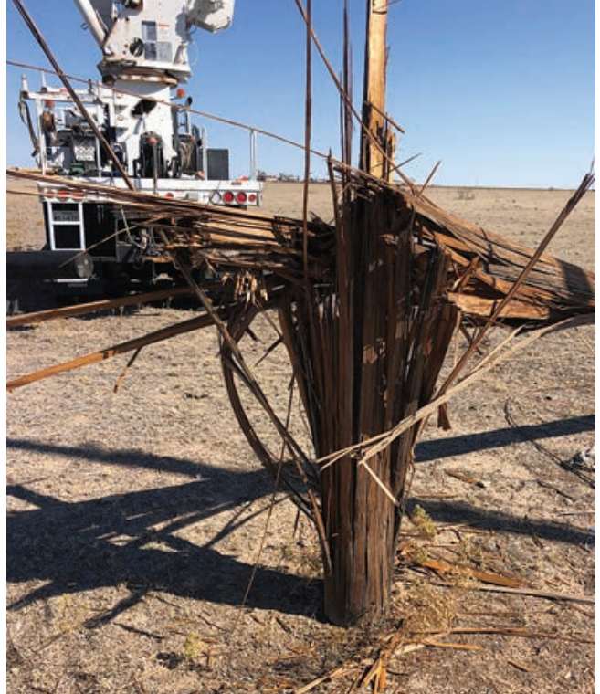
From August through October, Texas lineworkers faced sweltering and then arctic conditions after hurricanes in the Gulf and an ice storm in West Texas and the Panhandle devastated co-ops' infrastructure.
